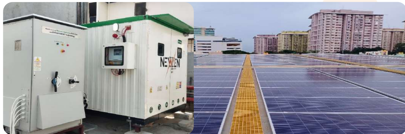
BESS Project Installation
